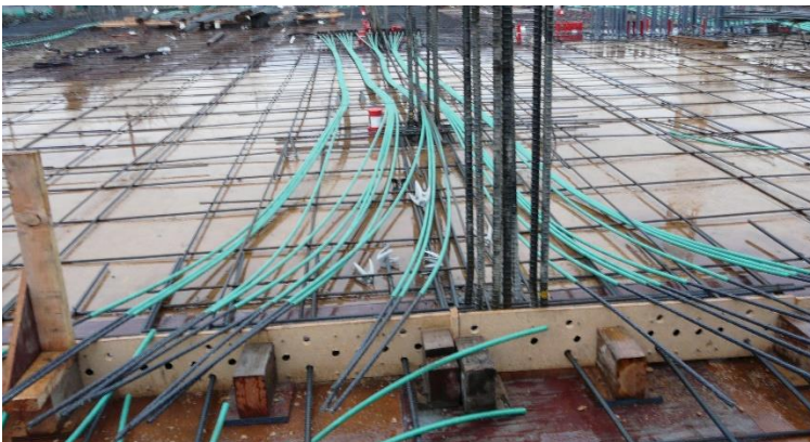
Post-tension cables
