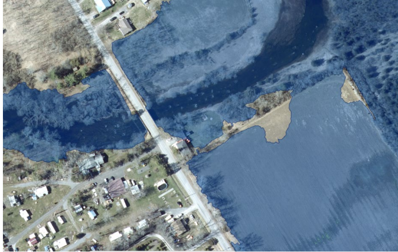
FIGURE 4-6: FLOODING UPSTREAM OF MELVILLE RD FOR THE 200-YEAR (0.5 % AEP) FLOOD EVENT
