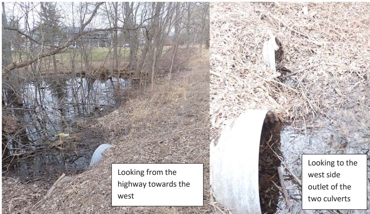
FIGURE 3-1: CULVERTS ALONG HWY 33-WEST SIDE OF THE ROAD
