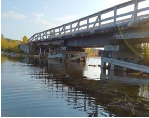
Photo 1: Upstream End of Structure
