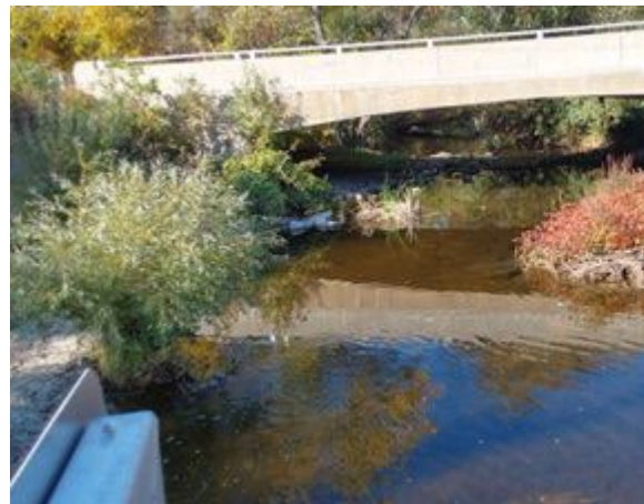
Photo 4: Looking Downstream from Structure
