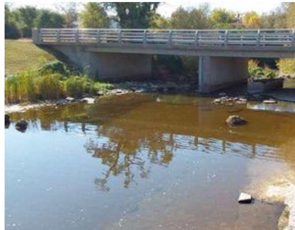
Photo 4: Looking Downstream from Structure
