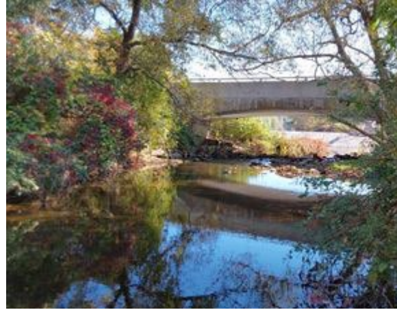
Photo 2: Downstream End of Structure
