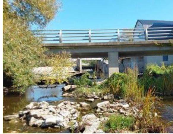
Photo 2: Downstream End of Structure
