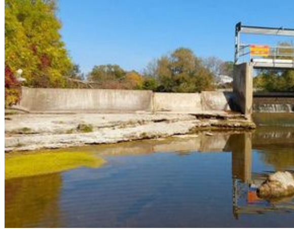
Photo 2: Downstream End of Structure
