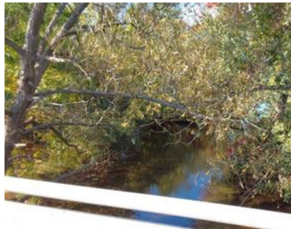
Photo 4: Looking Downstream from Structure
