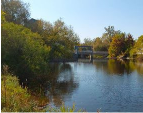
Photo 1: Upstream End of Structure
