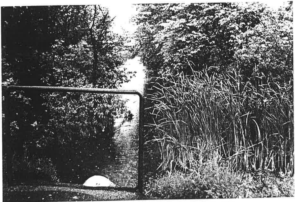
#8 - AT POINT A ON EAST SIDE LOOKING EAST
