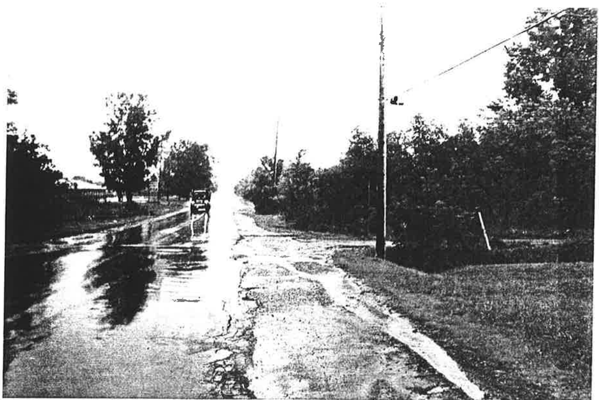
#2 - EAST SIDE LOOKING NORTH
