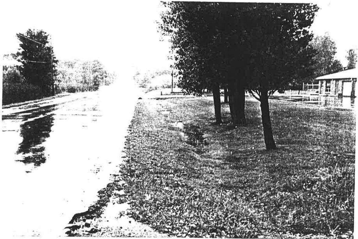
#1 - WEST SIDE LOOKING SOUTH
