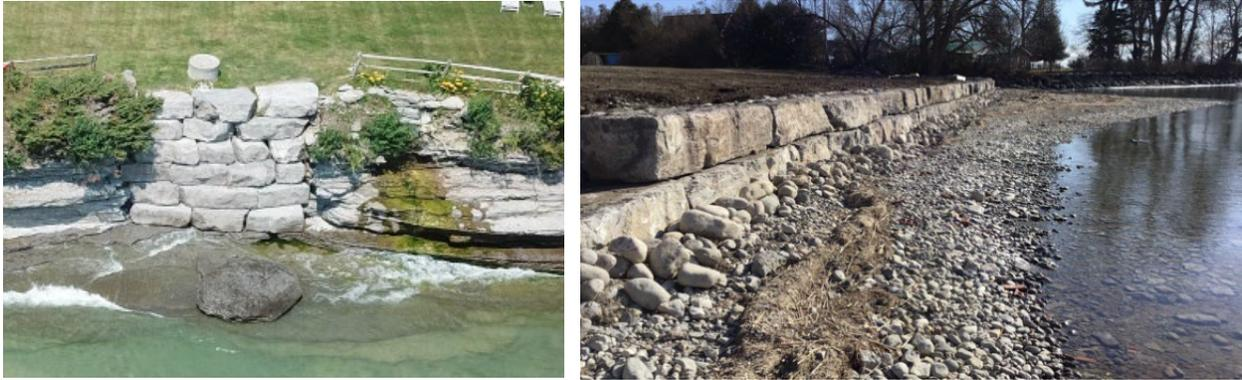
**Figure 7.12 Stacked armour stone seawalls on Lake Ontario, “plugged” into an eroded section of bedrock cliff (left) and at the back of a cobble beach (right).**
