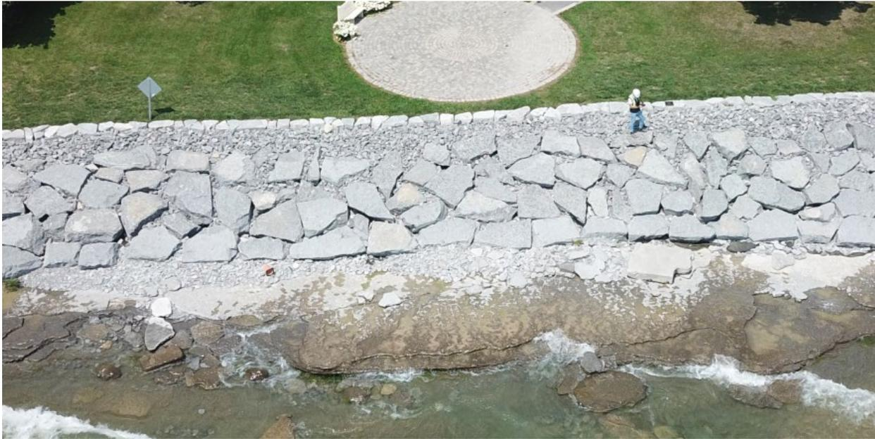
**Figure 7.11 Single-layer blocky armour stone revetment with toe stones “keyed” into underlying bedrock shelf**
