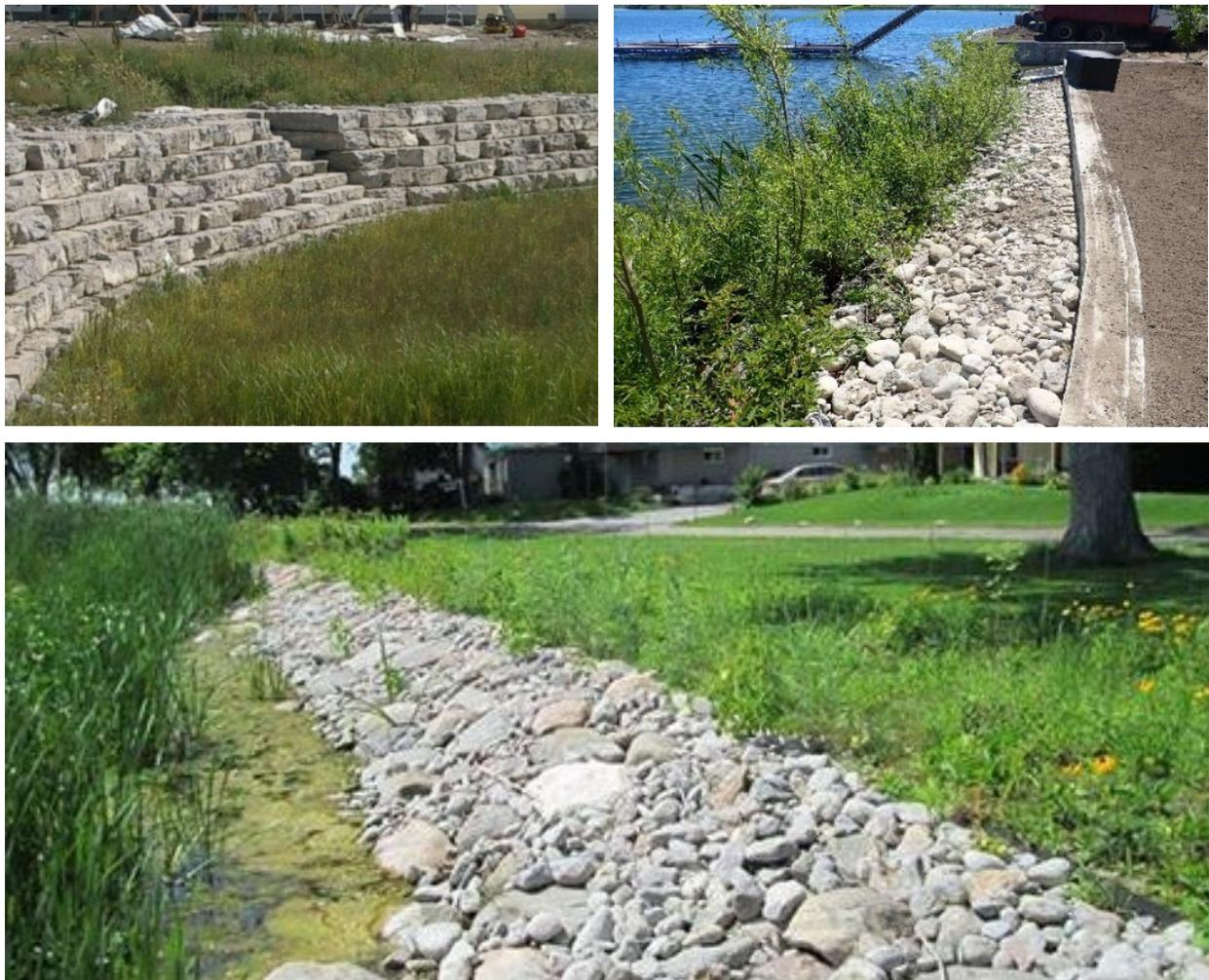
**Figure 7.15** Examples of hybrid grey/green shoreline protection schemes suitable for low exposure, low-energy shoreline environments such as those present in sheltered embayments and the Bay of Quinte
