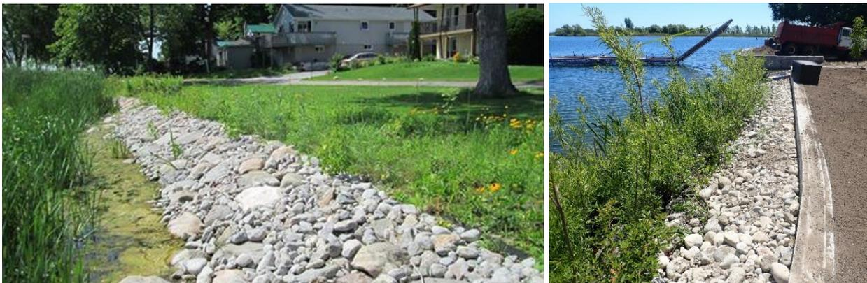
**Figure 7.8 Hybrid grey-green shoreline protection structures featuring stone and/or concrete infrastructure fronted by vegetated natural buffers and natural riparian conditions**
