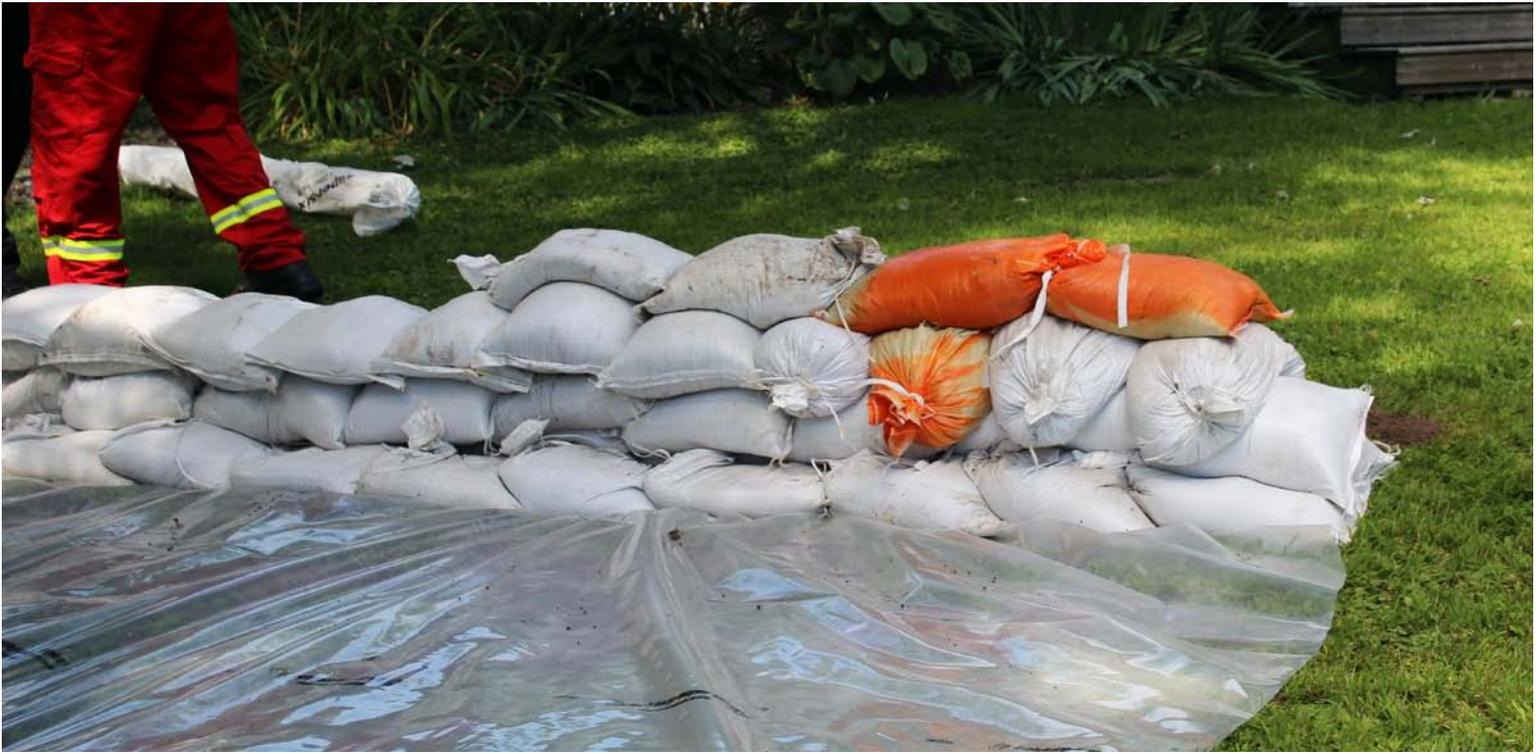
*Sandbagging is a simple and effective way to prevent or reduce flood water damage. It provides a barrier from flood water, protecting your property and home. In this document you will learn more about sandbagging and the safe and proper way to create a sandbag wall.*
