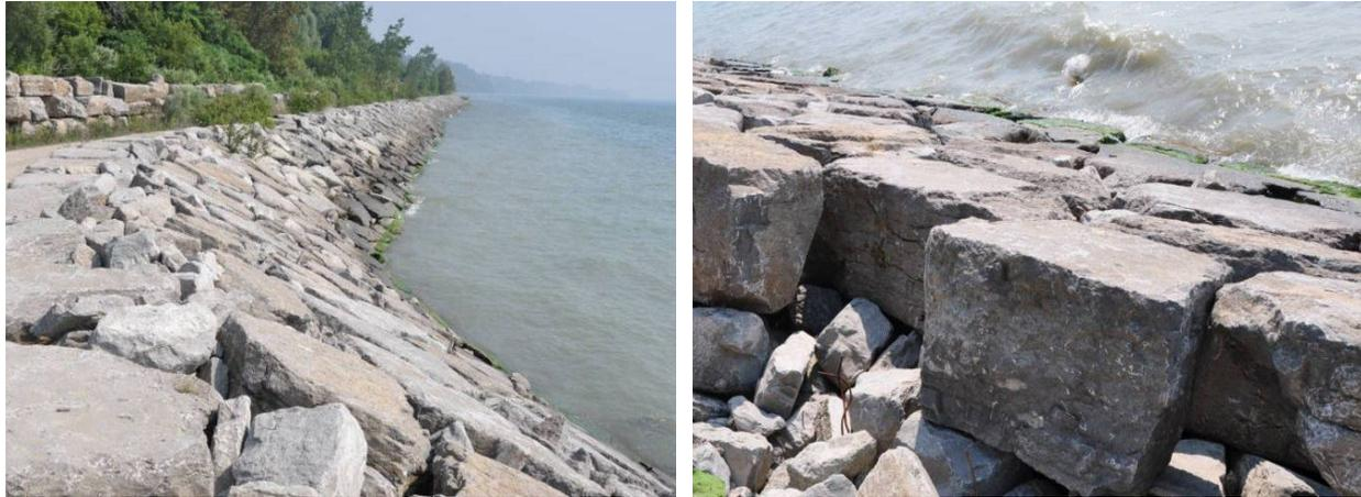
**Figure 7.9 Examples of single-layer, blocky armour stone revetments on Lake Ontario**
