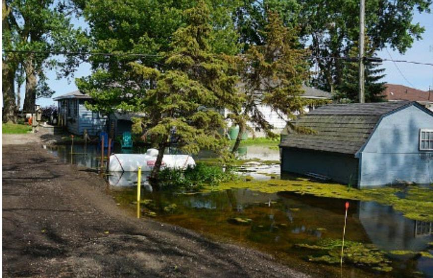
**Figure 5.6 Sewage ponding from failed septic systems caused by flooding in 2019 in the Marentette community, Southeast Leamington, Lake Erie**
