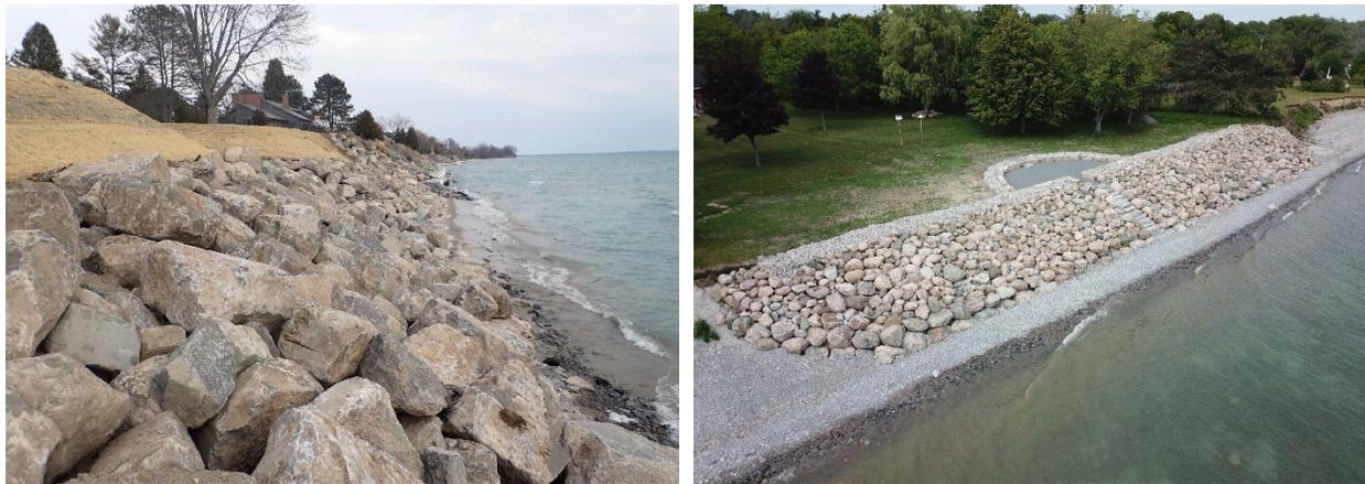
**Figure 7.10 Examples of conventional, randomly placed armour stone (left) and field stone (right) revetments on Lake Ontario**
