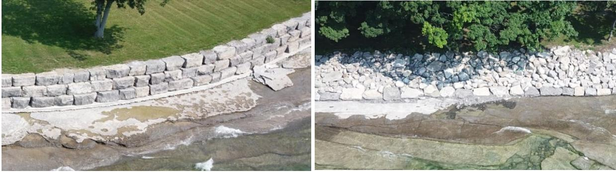
**Figure 7.6 Example of conventional shoreline protection structures on bedrock shorelines; stacked armour stone seawall (left) and “keyed-in” armour stone revetment (right)**
