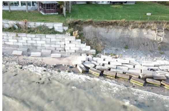
A significant advantage to sloping structures is that they tend to have gradual failure mechanisms such as displacement of structure elements (typically stones) or settlement over relatively long periods of time. By contrast, vertical structures tend to fail abruptly and catastrophically during a major storm event. Sloping structures can be monitored and maintained more readily throughout their design life relative to their vertical protection.
