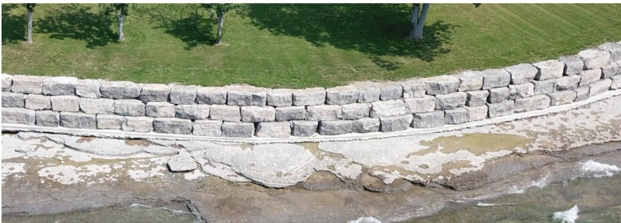
**Figure 7.13 Stacked armour stone seawall founded on a thin concrete foundation over an irregular bedrock shelf**
