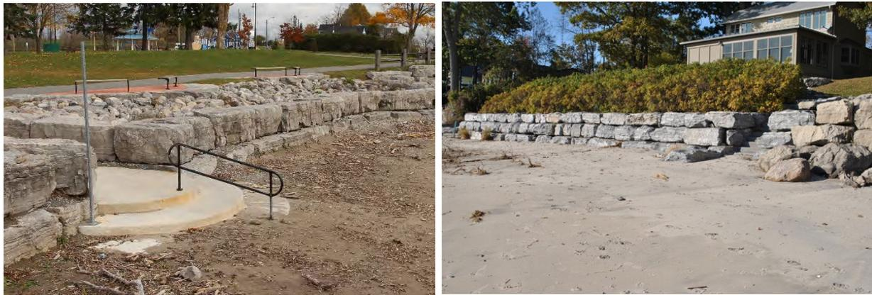
**Figure 7.16 Examples of stacked armour stone beach curbs**
